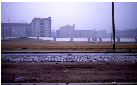
(c) Berlin's wall: M-Bahn as a technical demonstration to Eastern Berlin
