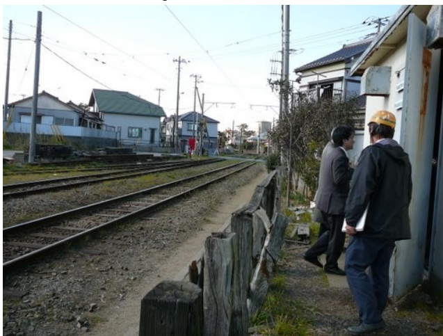
(b) The unique substation of Choshi Electric Railway
